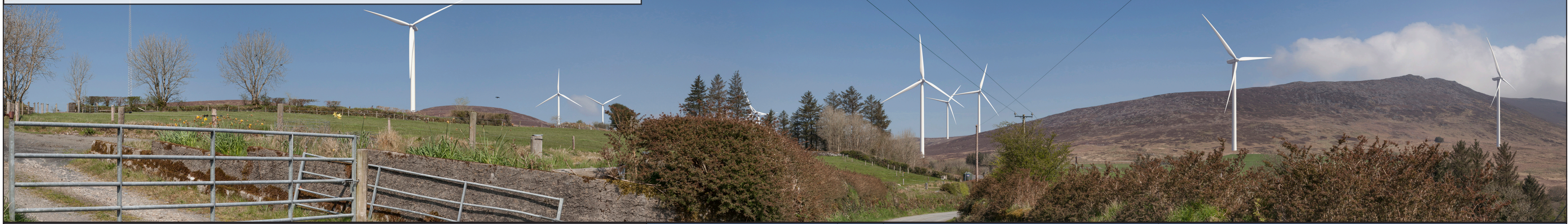
Option 3: Vesta V117 - 14 Turbines: Hub Height: 91.5m, Rotor Diameter: 117m, Tip Height: 150m.
