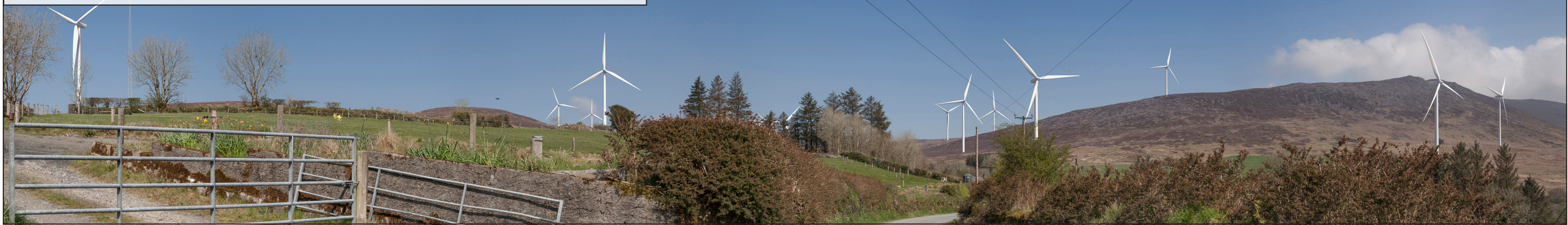
Option 3: Vesta V117 - 14 Turbines: Hub Height: 91.5m, Rotor Diameter: 117m, Tip Height: 150m.
